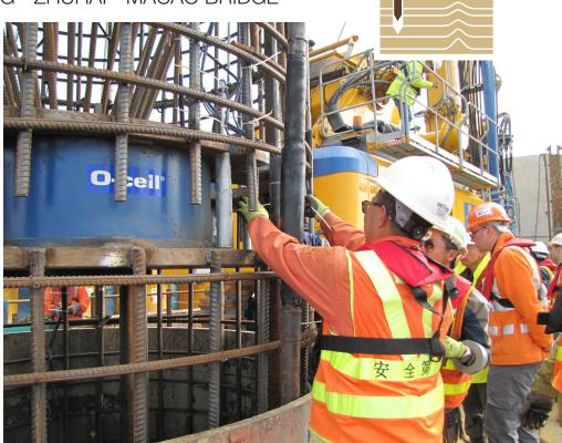
Inspection of loading assembly before cutting Osterberg Cell protection straps required during cage lifting operation
