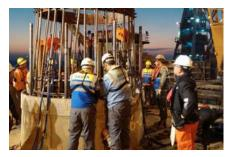
Preparation being carried out to protect Osterberg Cell instrumentation before lowering cage to final elevation
